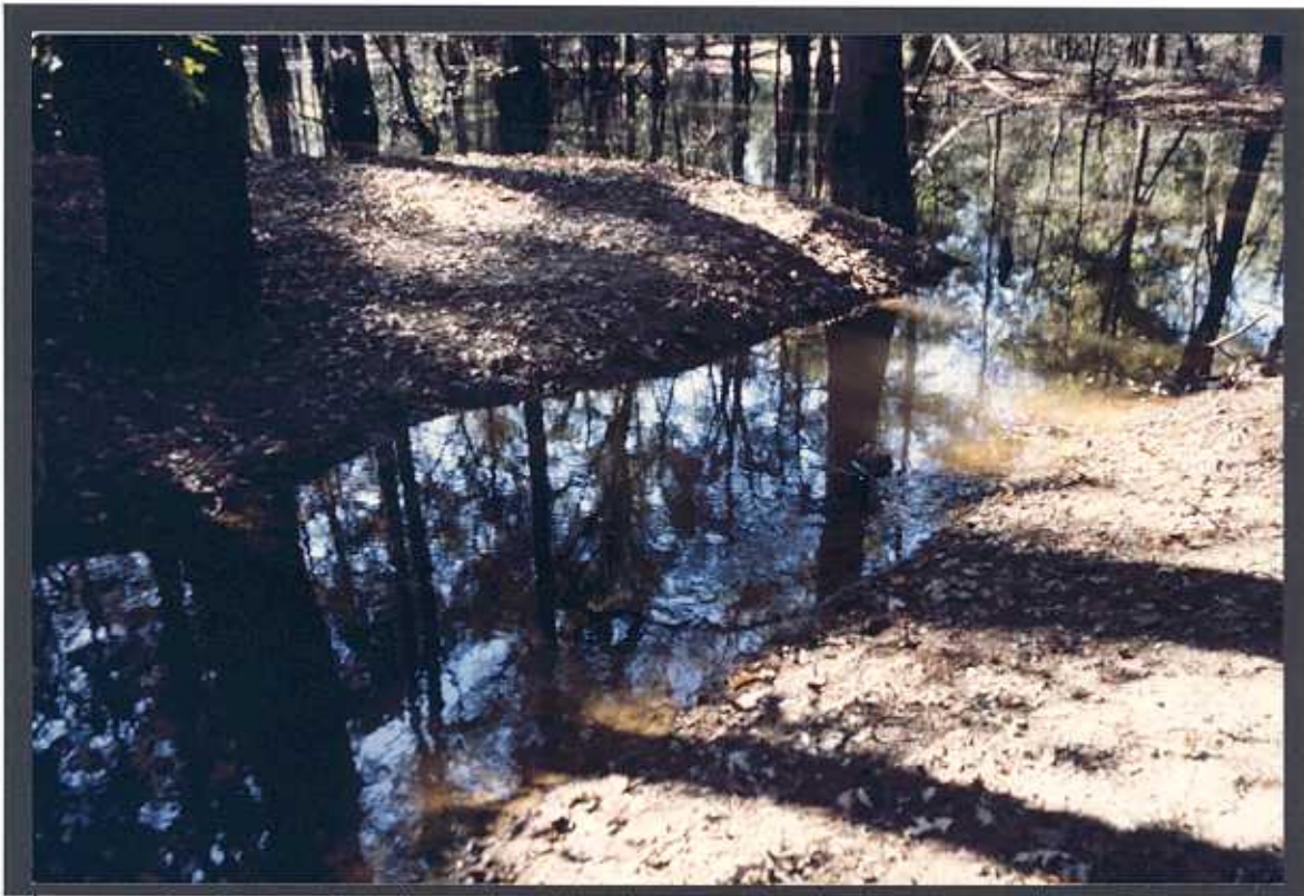
Figure 6. Breach of natural stream bank levee, Big Cypress Bayou, Texas.
