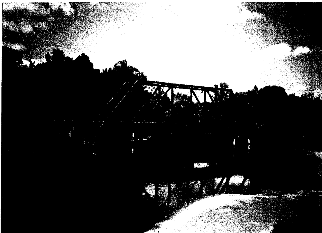
Photo 4. Historic railroad bridge located in Core area.
